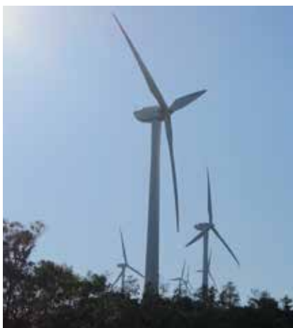
At the wind farm
